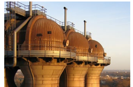
Blast furnace / stove dome
