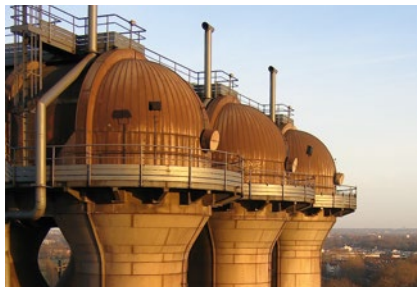
Blast furnace/Hot-blast stove
